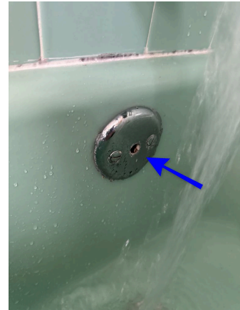
Copper is nonfunctional with a missing handle noted
