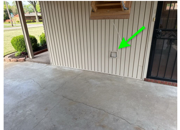
Dryer vent is located under the carport
