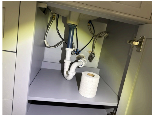
Under sink view
