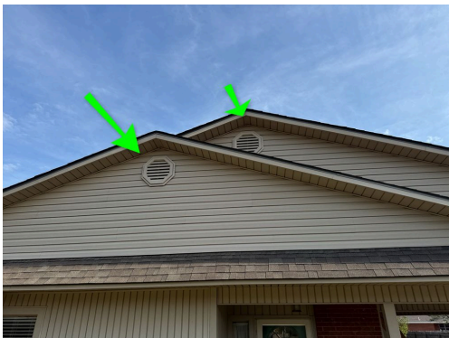
Gable vents noted
