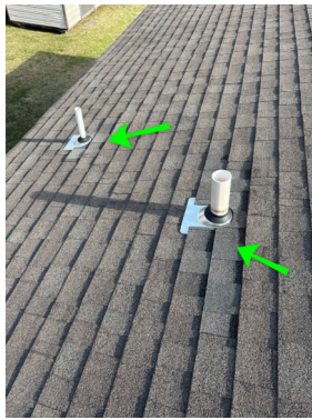
Couple of areas show repair or shingle replacement. Typical north facing fungal growth type staining noted
