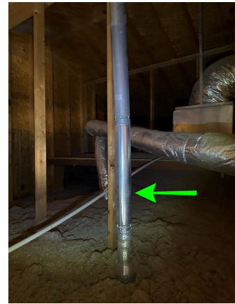
Double wall vent pipe is noted in the attic space.
