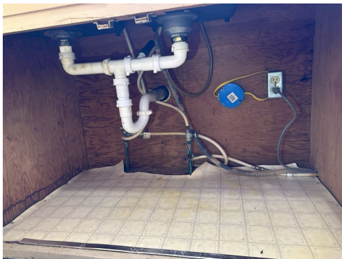
Under sink, View
