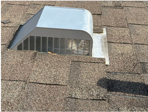
Roof vent, View
