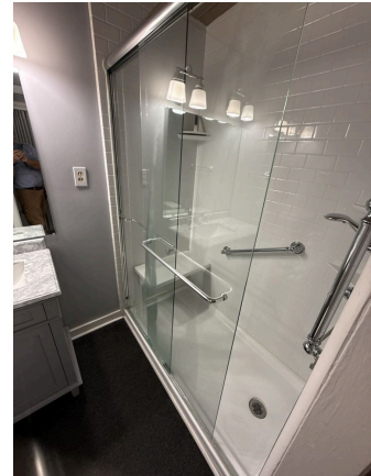
Shower enclosure appears functional
