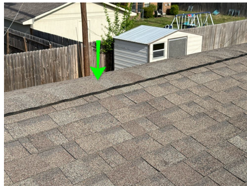
Ridge venting noted
