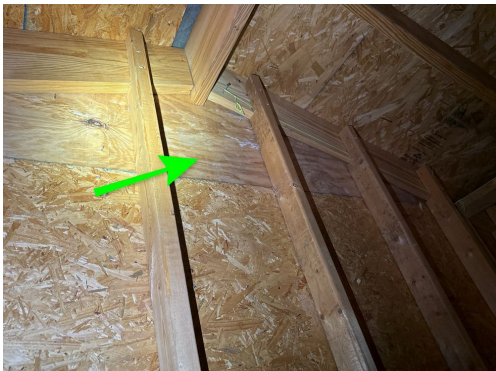
Gable event is not visible inside the attic space
