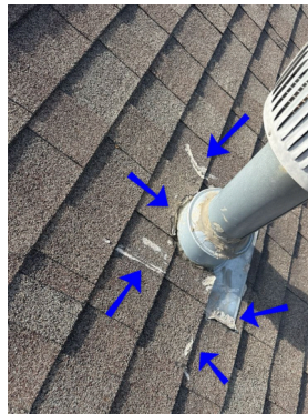
Sealant noted at a gas pipe penetration area
