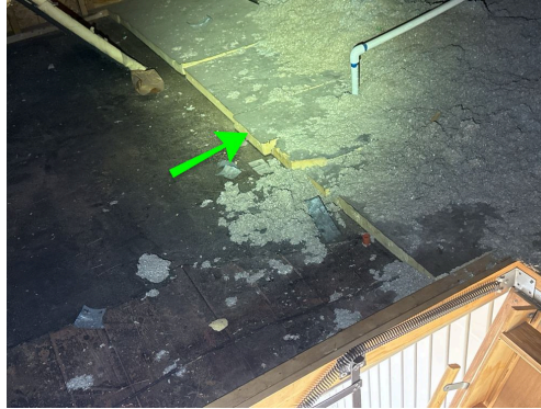
Insulated foam board is noted in areas.
