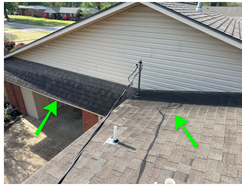
Couple of areas show repair or shingle replacement. Typical north facing fungal growth type staining noted
