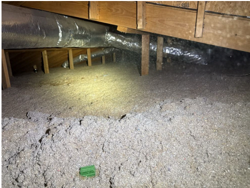
Limited view into the North attic section.
