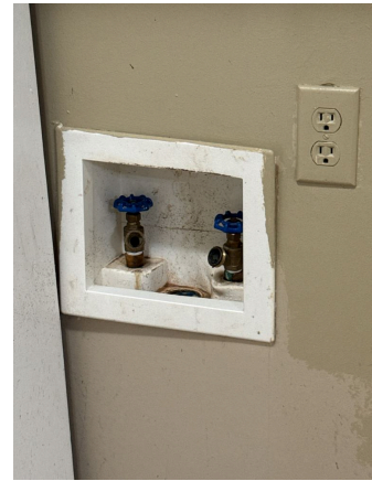
Water valves are not marked hot and cold.
