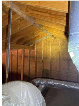
South framing view.
