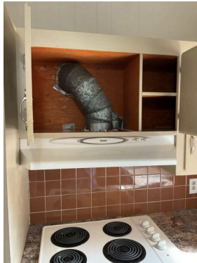
Vent pipe view
