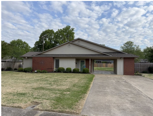
South facing view
