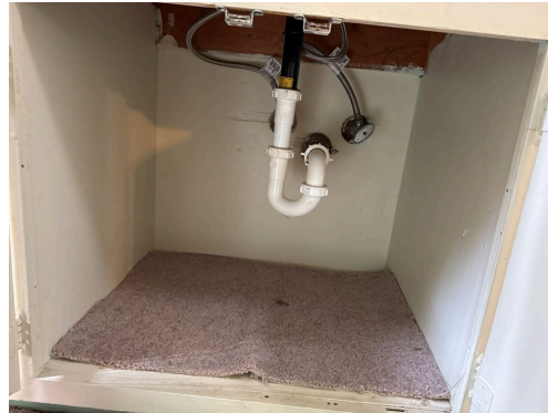
Under sink view
